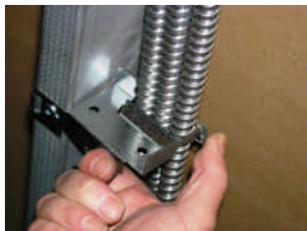
Bend side locking tab
