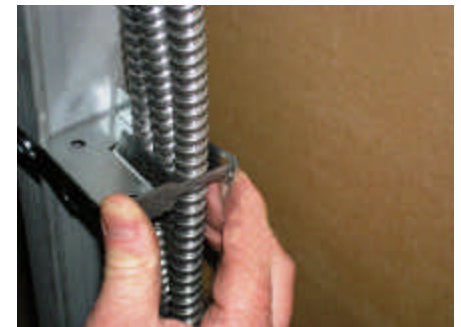
Engage back tab with locking tab
