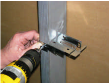
Attach to stud using SMS8 screws or equivalent
